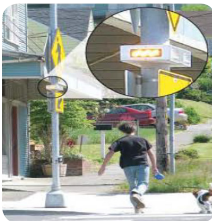
RRFB with Pedestrian Verification Light
